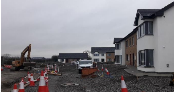
Construction Works at Station Avenue Phase 2 – Ballyragget – Jan 2021
