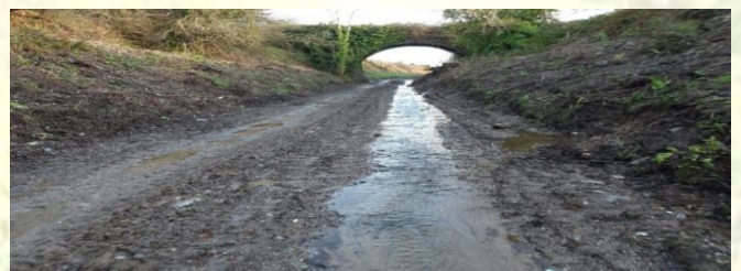
View of track near Bellfield following clearance
