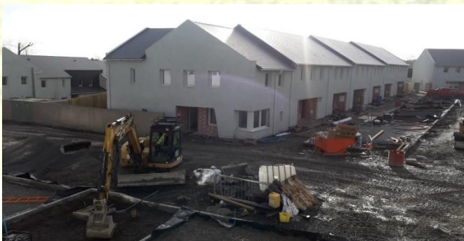
Construction nearing completion – Glebeside, Castlecomer – January 2021
