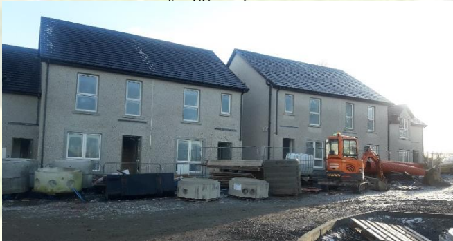
Blackwater Grove, Kilmacow – under construction January 2021
