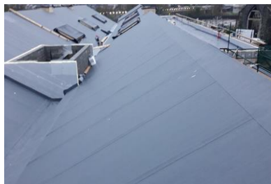
Installing frames of Roof lights commenced.
