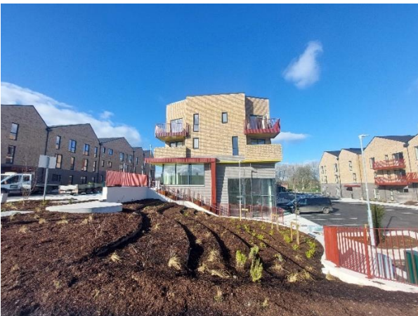
Croker's Hill Housing Scheme- Community Centre incorporated into the build
