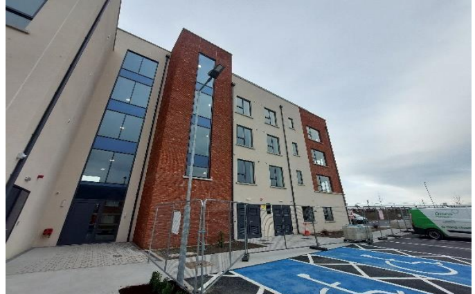
Castleoaks - 30 Apartments Turnkey and Part 5 - Handed over February 2025
