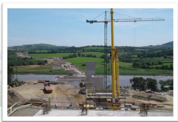
Barrow Bridge – Pink Rock piers rising towards deck soffit level
