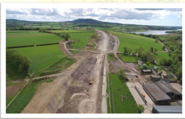
Earthworks on Glenmore side with Pink Rock in background.
