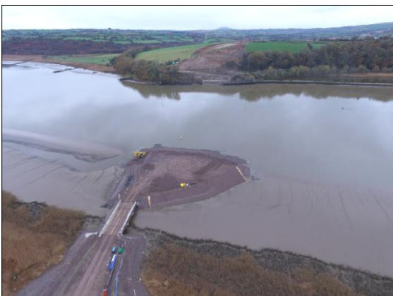
Barrow Bridge - Temporary Impermeable Working Area for Pier 4
