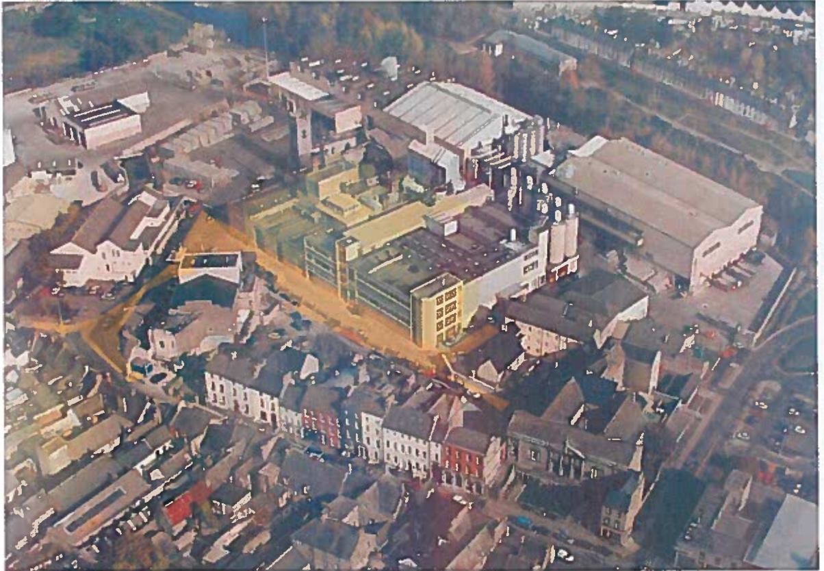
Aerial View of Site from South West
