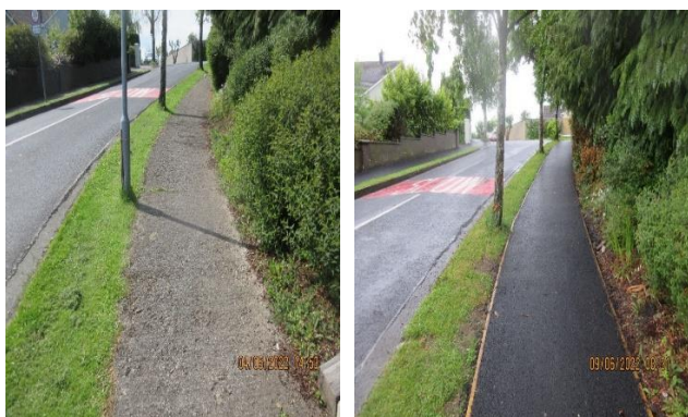
Footpath Repairs At Glendine Before & After
