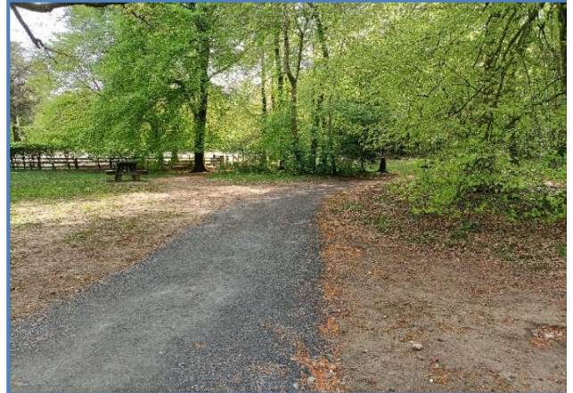
Improvements to footpaths underway in Woodstock
