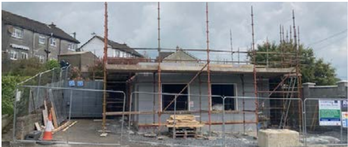
Work Progressing on 2 units in Graiguenamagh – infill scheme – ICF construction
