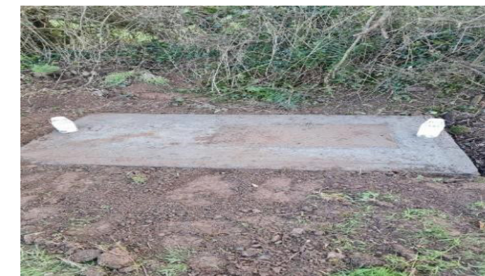
New Cover provided to existing Septic Tank following inspection
