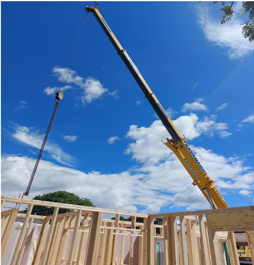
Erection of timber frame at Inchacarron Mullinavat. Low Carbon Construction
