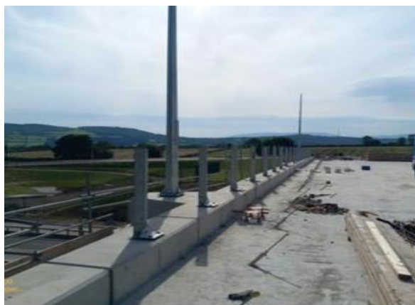
Bridge Parapet & Public Lighting Installation
