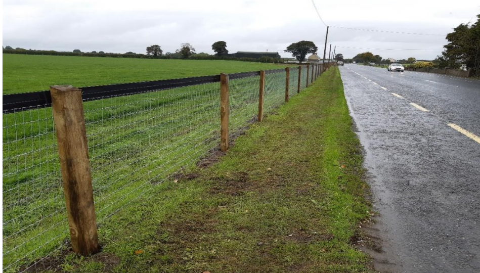
Typical Fencing Retrofit completed works on the N10 Dundaryark
