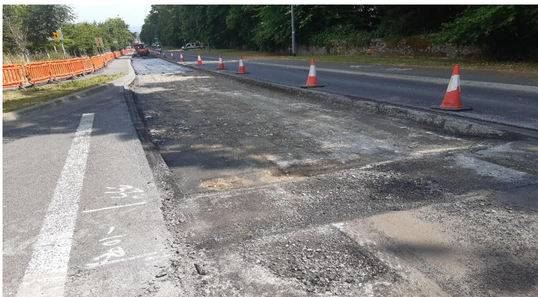
N76 Callan Road, Kilkenny. (Reconstruction Works in progress)
