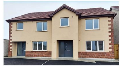
17 UNITS AT LIMEGROVE, FERRYBANK
