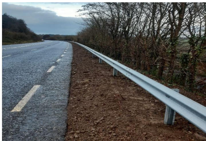
New Section of VRS on the R723 (Former N25)
