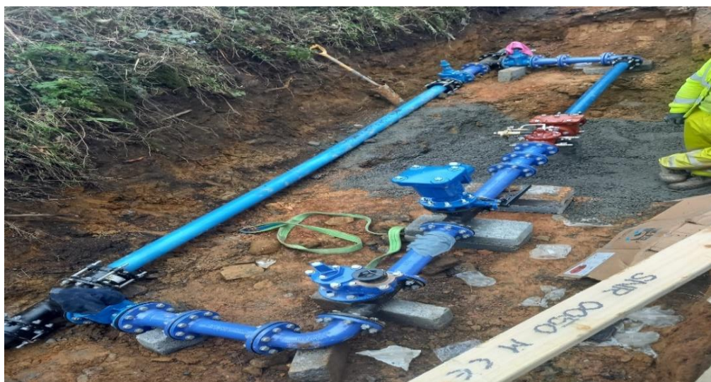
PRV installation at Kiltown Cross, Inistioge
