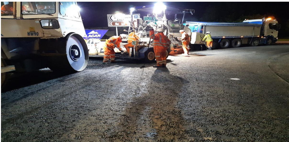
Typical Night Works underway by Contractor on N10 Dublin Rd Roundabout
