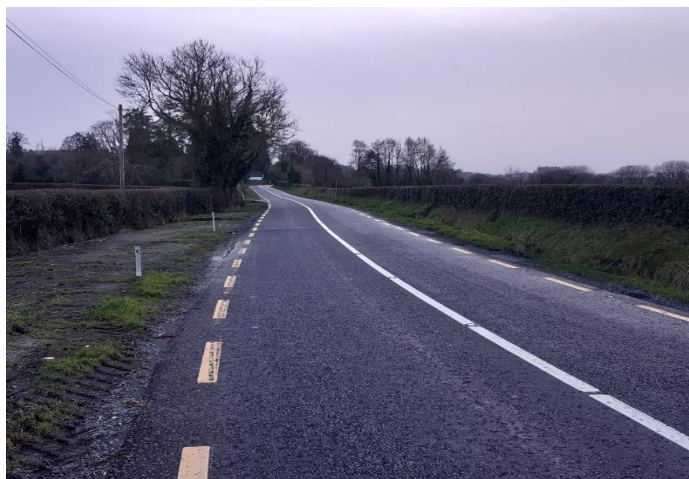
N78 Webbsborough – Finished Pavement
