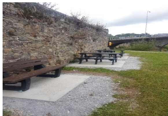
Clean up at Thomastown Bridge
