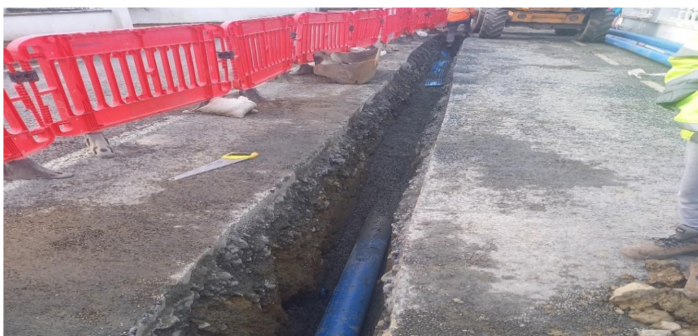
Construction of new water-main at Knocktopher Village
