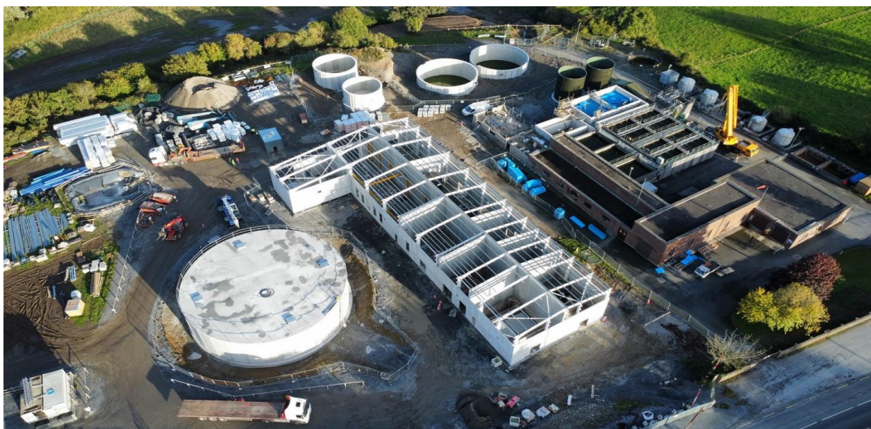
New Chemical Building & Tanks – Kilkenny City RWSS Troyswood
