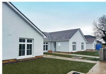
5 UNITS, BERKELEY DRIVE, FERRYBANK
