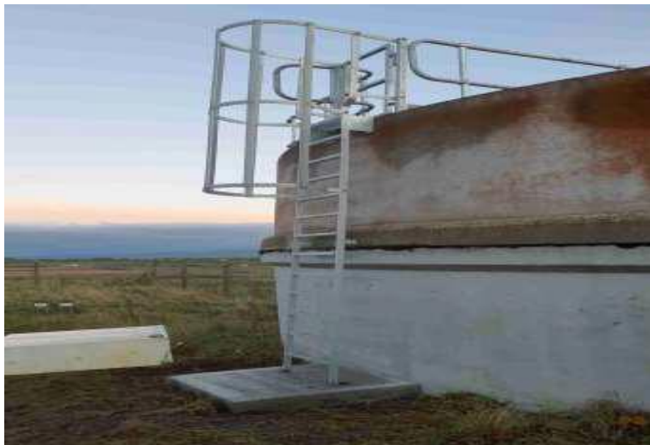
New Access Platform with Handrail support at Galmoy WWTW
