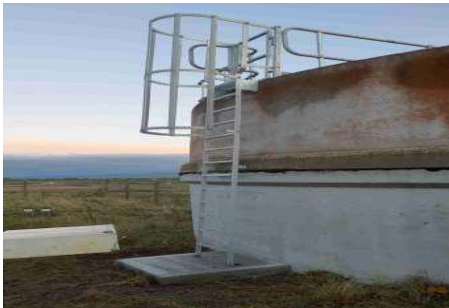
New Access Platform with Handrail support at Galmoy WWTP
