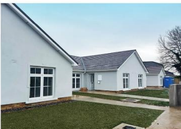
5 UNITS, BERKELEY DRIVE, FERRYBANK
