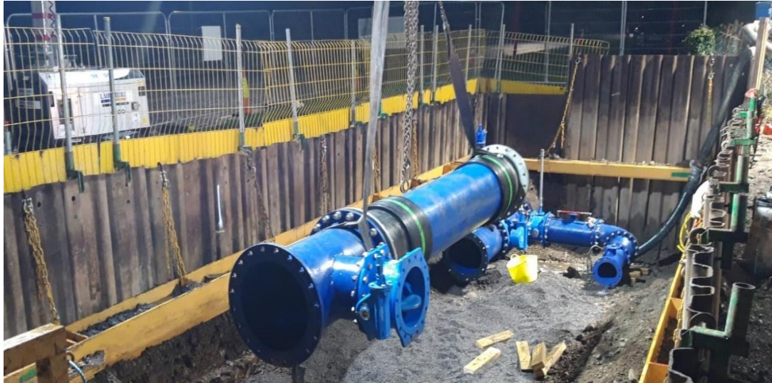
Installation of PRV in Kilkenny City February 2021
