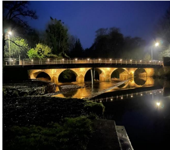
Night View of Footbridge
