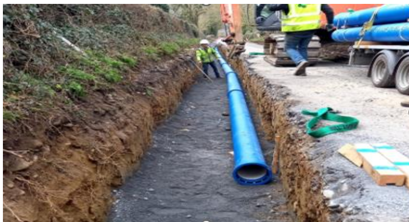
Construction of Ductile-Iron Rising Main Norelands WTP - Rathduff Reservoir
