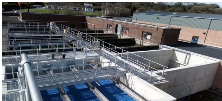
Kilkenny City RWSS – New Clarifier & Rapid Sand Filter
