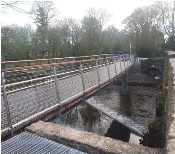
View of New Footbridge
