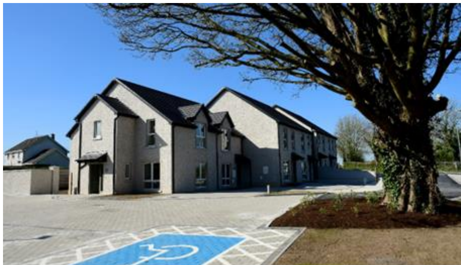
Blackwater Grove, Kilmacow, 16 units 2021 – Turnkey
