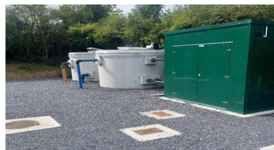
Disinfection Programme works at Gorteen WTP
