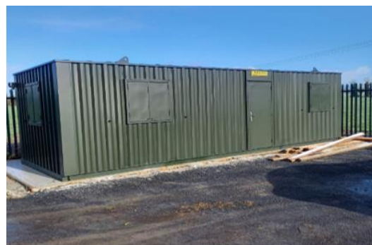
New Welfare Facility installed at Loon Water Treatment Plant
