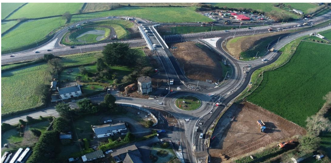
Overhead drone footage of the compacted grade separated junction.
