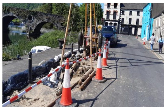
Site investigation works at The Quay, Graiguenamagh
