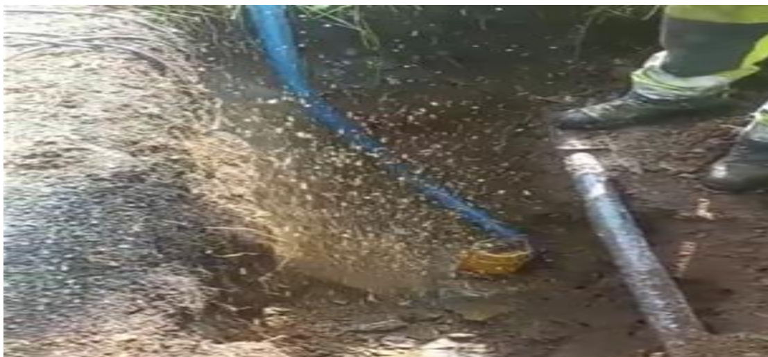
Find & Fix Leak repair at Kilcross, Inistioge
