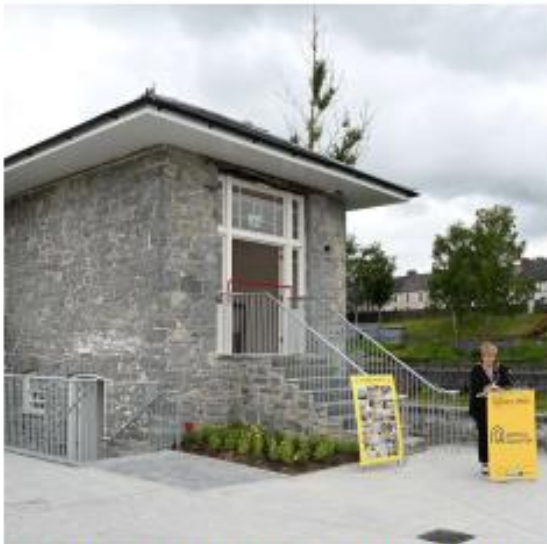
OFFICIAL OPENING OF THE RESTORED TEAHOUSES
