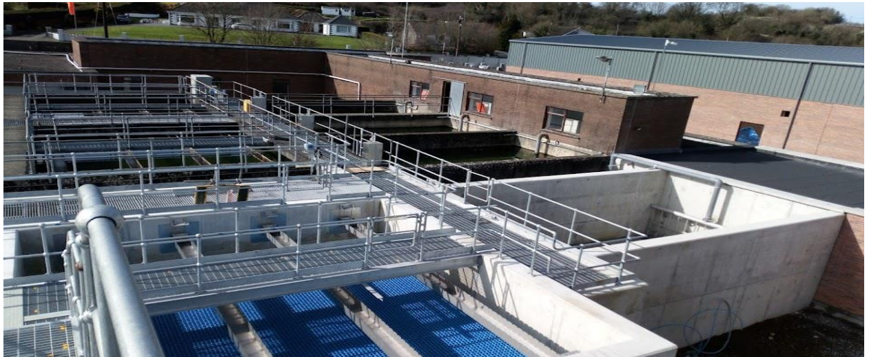
Kilkenny City RWSS – New Clarifier & Rapid Sand Filt
