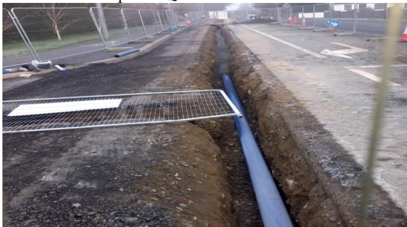
Construction of new HDPE watermain at Dublin Rd, Thomastown
