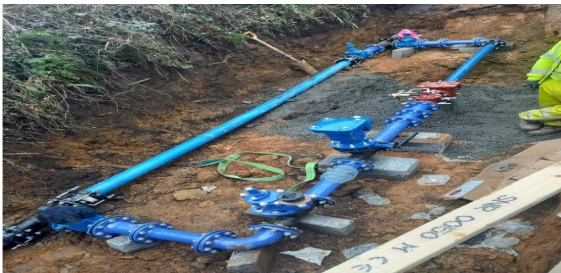
PRV installation at Kiltown Cross, Inistioge
