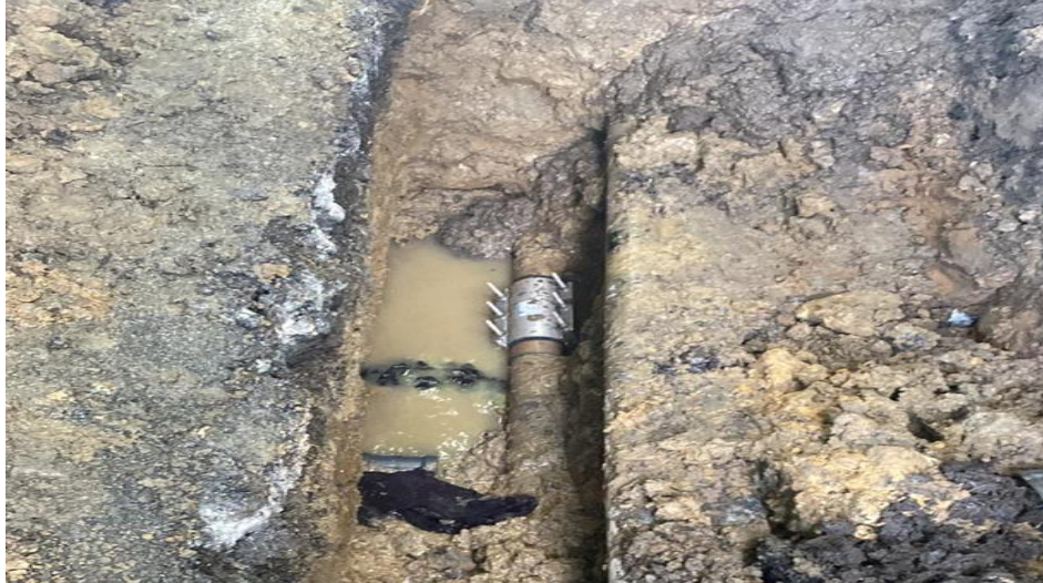
Find & Fix Leak repair at Kilcross, Inistioge
