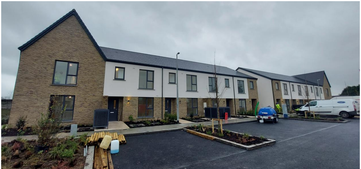
College Park Crescent – 10 x 3 bed houses completed November 2024
