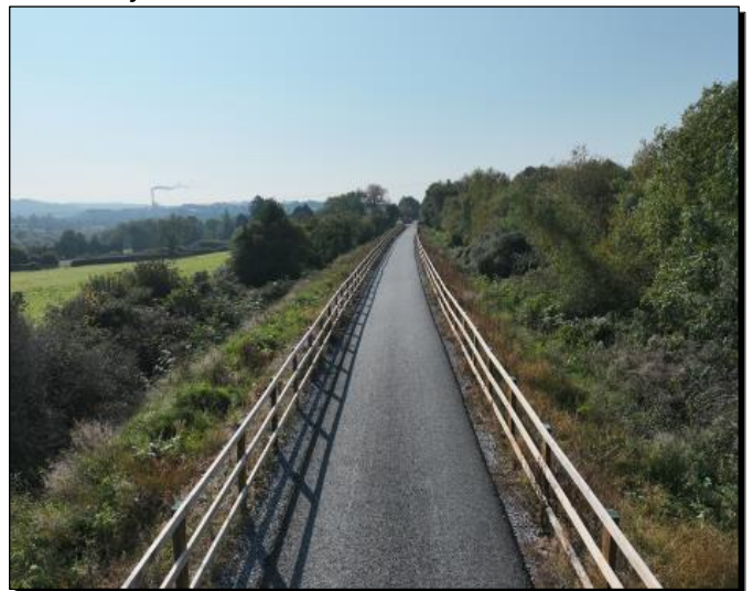
Final Pavement Overlay
