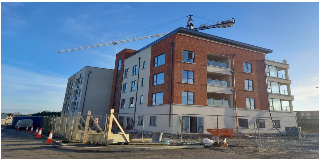
The Rise, Castleoaks, Kilkenny – 30 apartments almost complete
