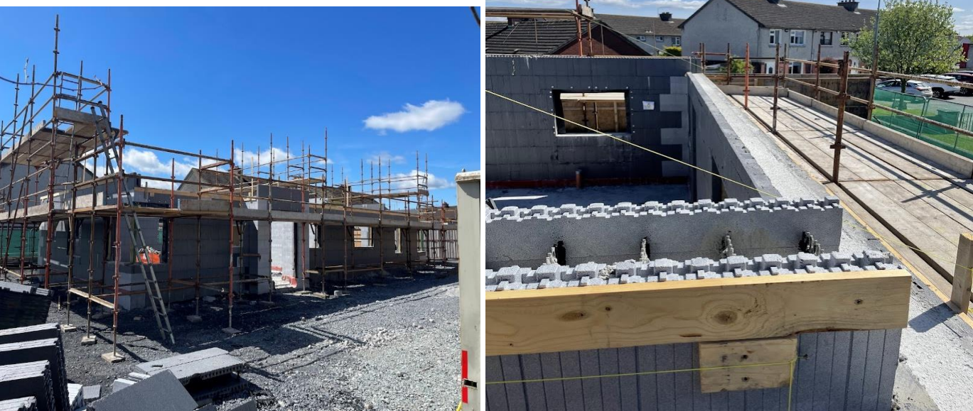
Construction of 2 Wheelchair Accessible Houses at the Old Community Center in Loughboy, Kilkenny The Houses are being constructed using Insulated Concrete Form (ICF)
