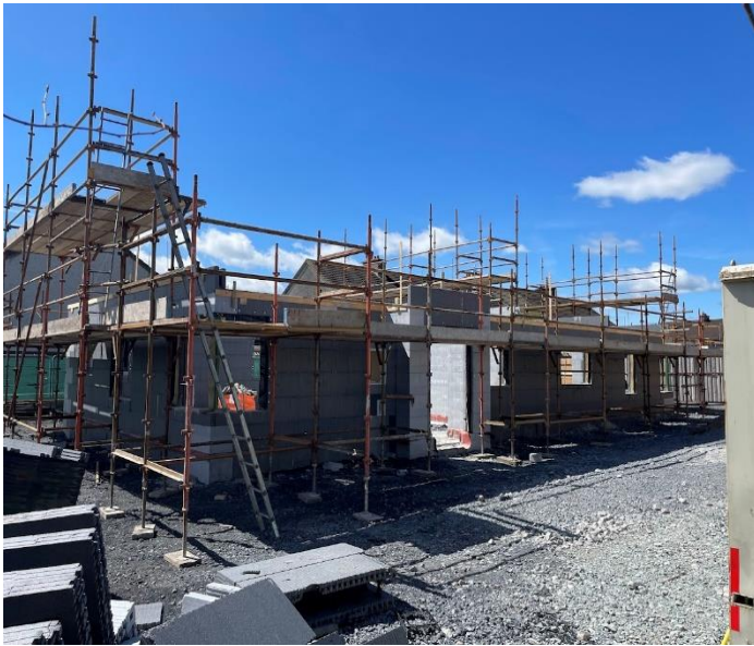
Construction of 2 Wheelchair Accessible Houses at the Old Community Center in Loughboy, Kilkenny The Houses are being constructed using Insulated Concrete Form (ICF)
