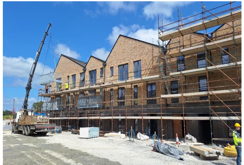
Construction of 2 Wheelchair Accessible Houses at the Old Community Center in Loughboy, Kilkenny The Houses are being constructed using Insulated Concrete Form (ICF)
