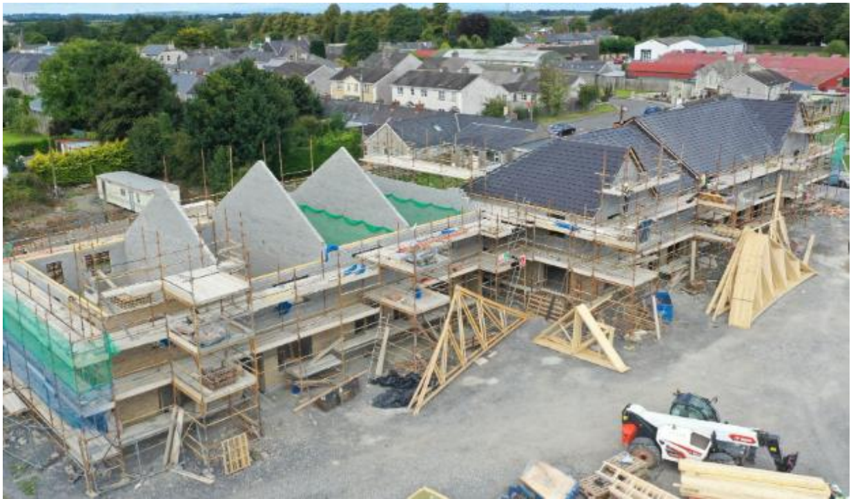
Turnkey Housing Project – 18 units on site at Ardreagh, Lumper Lane Urlingford.
