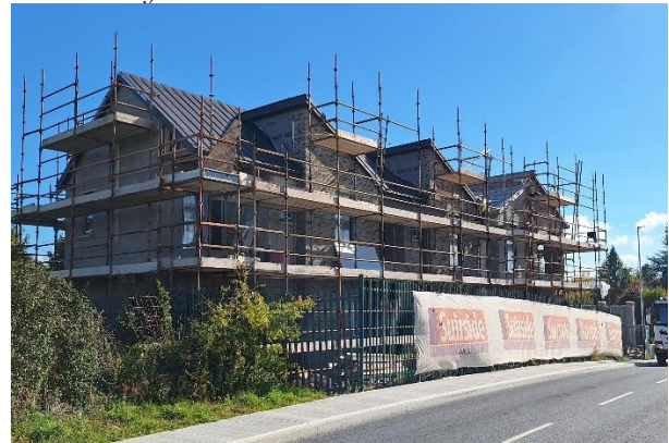
Construction of 6 social apartments at Teach Aimsire, Dunningstown Road, Kilkenny due for completion in March 2026
