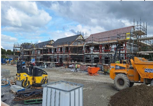
Construction of 20 social units including a group home at An Tobar, Freshford due for completion in July 2026
