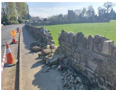
Wall repairs in progress
