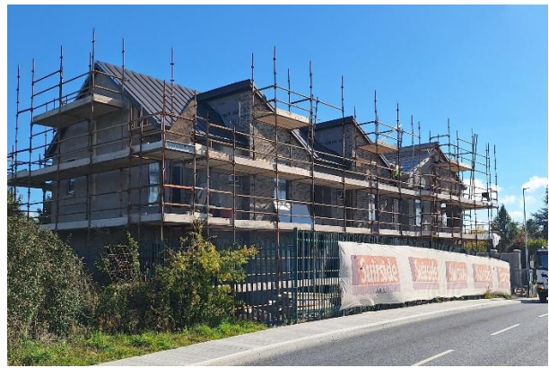
Construction of 6 no. social apartments at Teach Aimsire, Dunningstown Road, Kilkenny due for completion in March 2026
