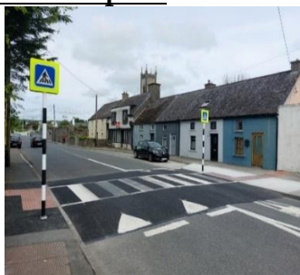
Installation of Pedestrian Crossing & ramps completed
