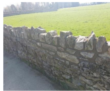
Wall repairs completed.
