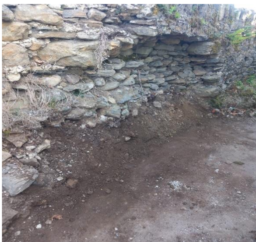
Wall Collapse at Cloghabrody
