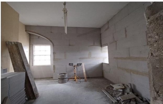
Before : Garda Station Back Office 2024 – Calsitherm Insulation
