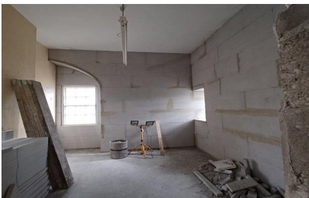
Before : Garda Station Back Office 2024 – Calsitherm Insulation
