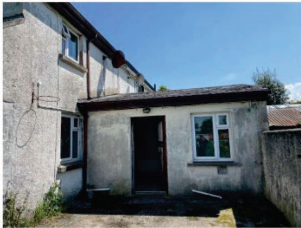
Rear Extension to be demolished
