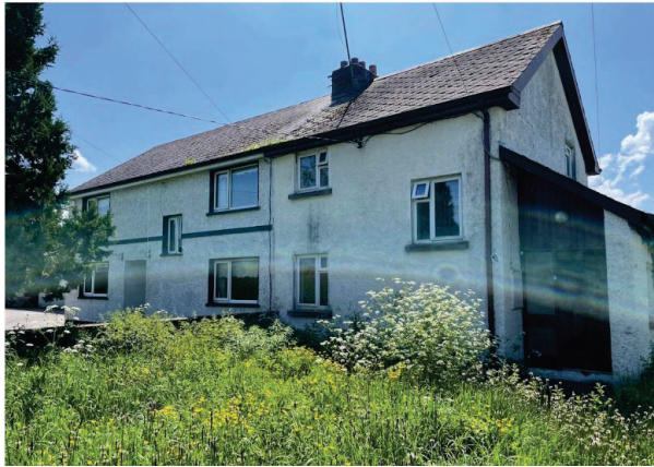
Front elevation of dwelling
