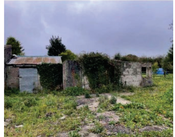
Rear Shed to be demolished
