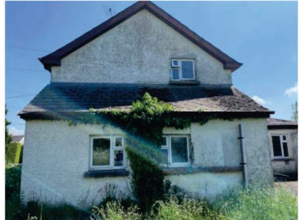
Side extension to be demolished
