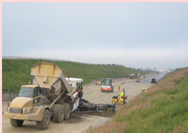
CBM Pavement Works North of Twomileborris
